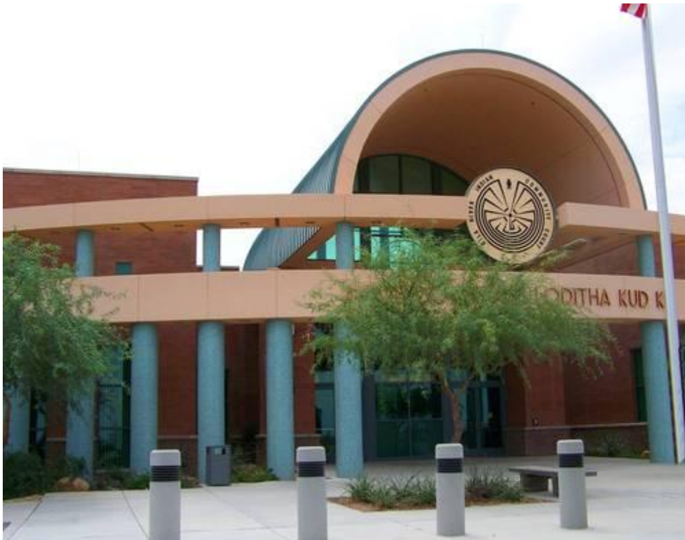
Gila River Indian Community Court House
